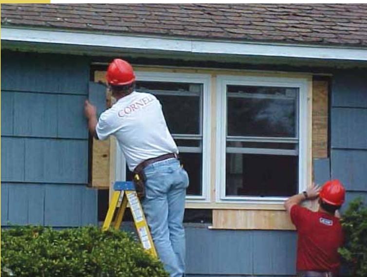
◀ Weatherization technicians repair and seal around windows
