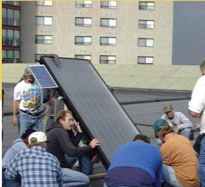
▲ **Crew installing a solar panel for a solar hot water system**
