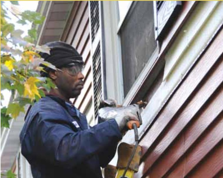
▲ **Weatherization technician drilling siding for sidewall insulation**
